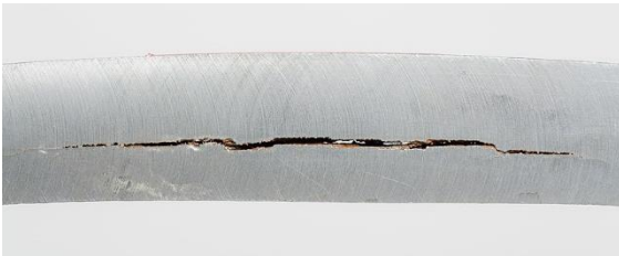
Hydrogen Induced Cracking
